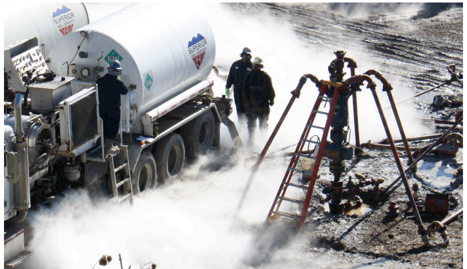
Wellhead setup used for foam fracs and gas fracs.
